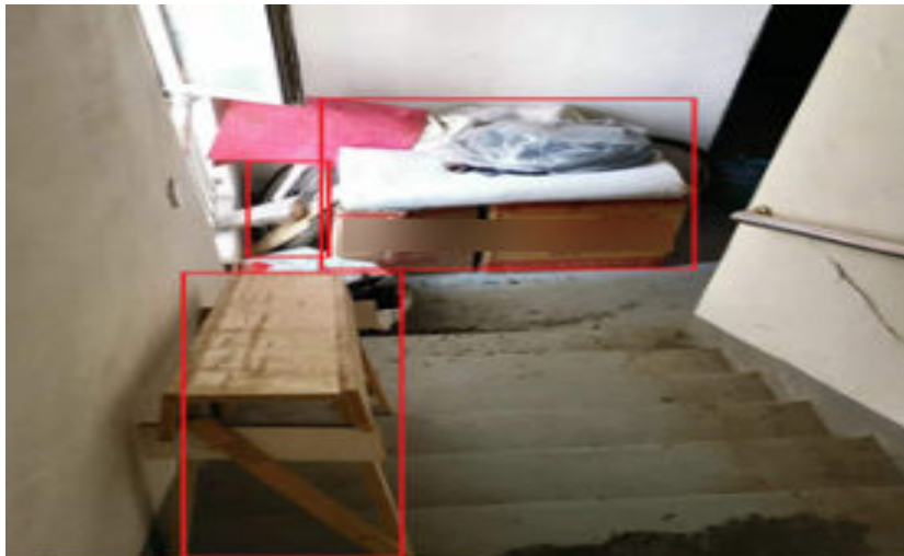
Figure 3-8 Detecting whether fire escapes are obstructed
