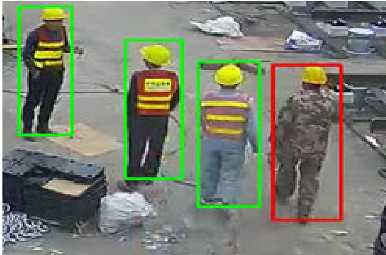
Figure 3-9 Safety helmet and reflective clothing detection
